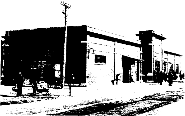
Above: B&MR Depot built during the early 1900s.
